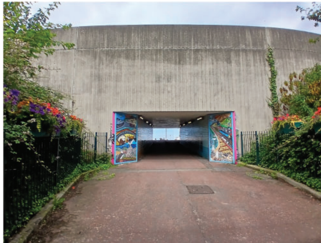
Fig. 12. Brutalist-style pedestrian underpass at Penmaenmawr from beach to town (image: J Paull).
